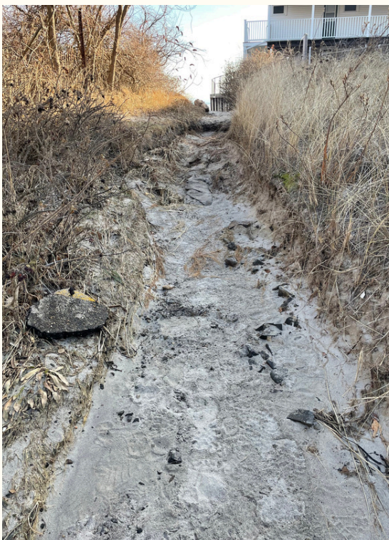
Condition of the access path after storms
