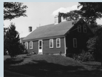
Goodale-Bourne Farm 412 North Village Road
